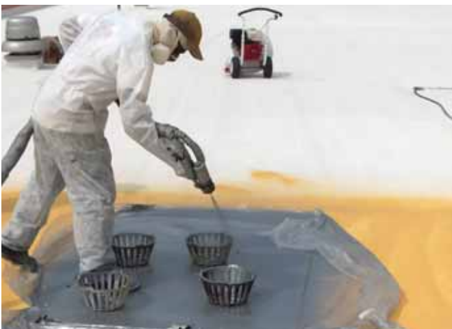
Any drain or vent covers were removed and individually coated with the VFI-540 aluminum polyurea elastomeric topcoat (left). When replaced on top of the drains, the protected covers seamlessly blended in with the rest of the roof.
