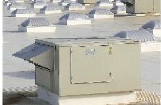
Conventional gas-fired rooftop heaters often have efficiency ratings between 78 and 82 percent. They are usually purchased with air conditioning units and provide both space heating and cooling in one system.
