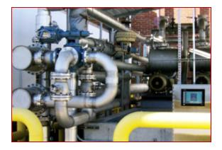
Based on recommendations from their Save Energy Now assessment, Shaw Industries in Dalton, Ga., installed a waste water heat exchanger on their Kuster dye line to capture excess heat, saving a significant amount of money and energy.
