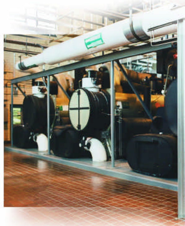
Above and right: Trane Duplex CenTraVac electric centrifugal chillers operate at exceptionally high efficiency and their low condensing water requirements allow the enlarged plant to continue to use the existing supply pipeline.
