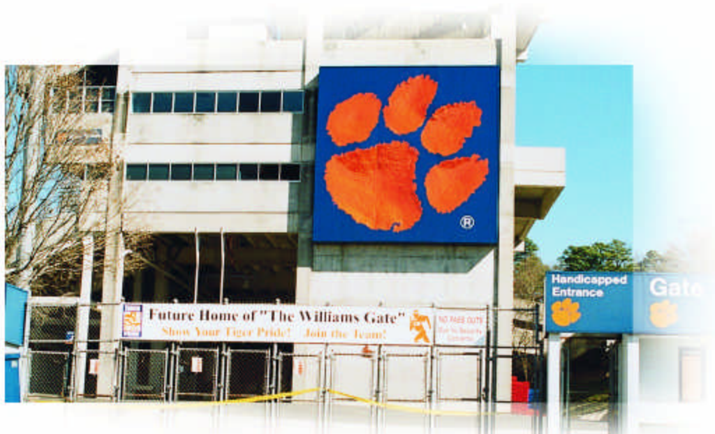
Condensing water is supplied by a pipeline that runs directly beneath the Clemson football stadium.
