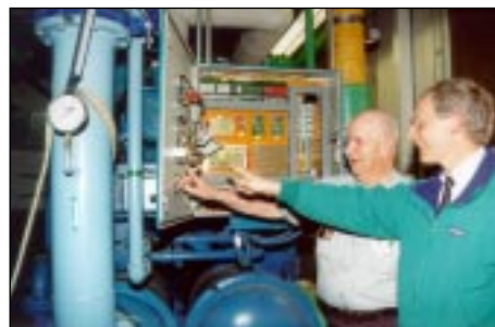
St. Elizabeth's Hospital, Chicago, as seen from its new OB/GYN wing (l.). Chief Engineer Dick Gilligan and Peoples Energy Product Specialist Mark Kruse (right) review details in the intricate Honeywell control panel, which monitors two 350-ton dual-engine TECOCHILL® chillers.
